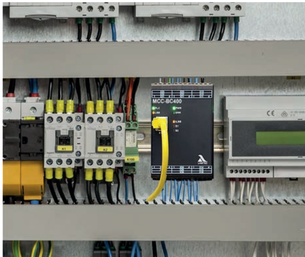
LAMTEC BurnerControl BC400 with control cabinet installation
