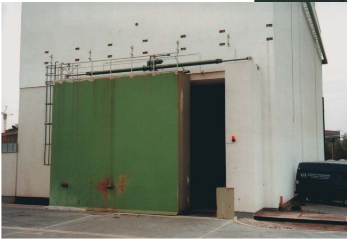
Gate actuator Force: 10 t, Stroke: 7000 mm
